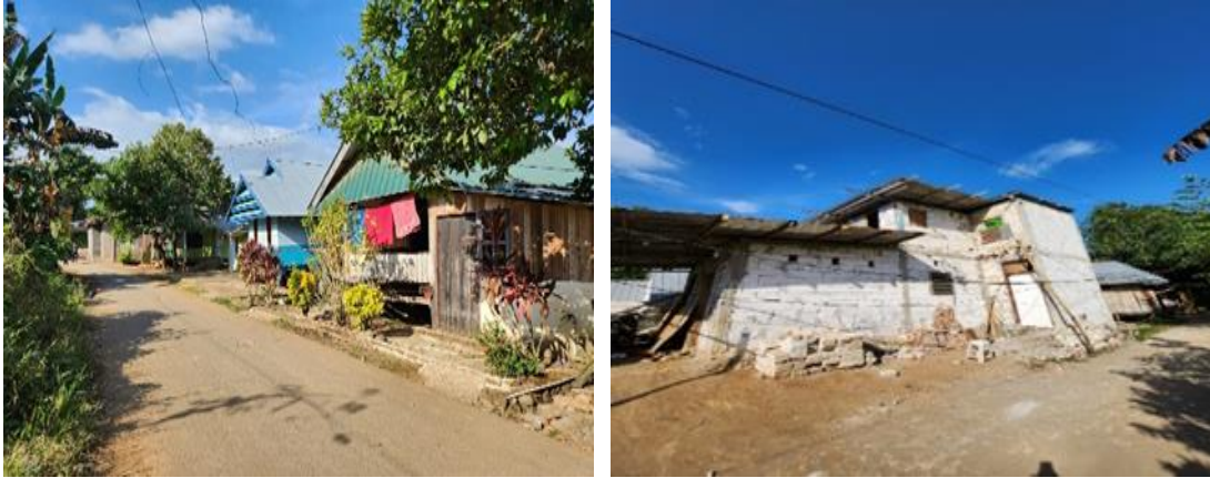
Figure 4. The House Condition of Jama'ah An-Nadzir Source: Field Survey, 2023
