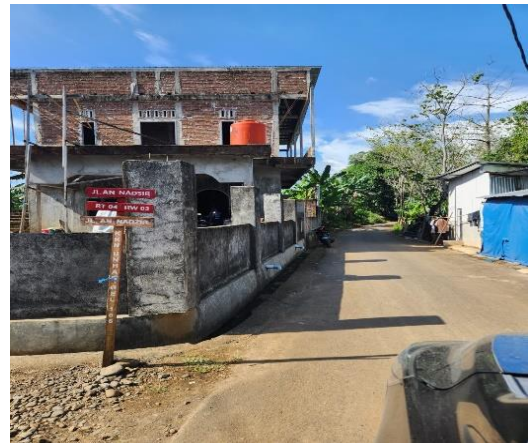
Figure 3. Condition of Surrounding Infrastructure Source: Field Survey, 2023
